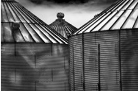
301. Grain Silo No. 20 $75 8X12 image (print only) Bin Location: BIN0
