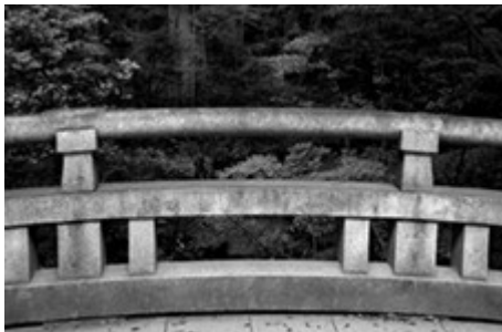
129. Foot Bridge No. 2
