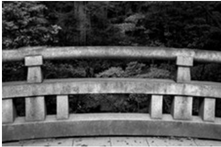
128. Foot Bridge No. 2
